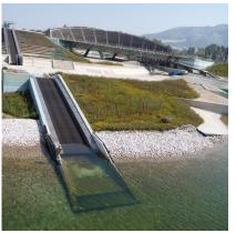
Optionally, the starting of the conveyor belt can be triggered by passing a boat in front of a radar detection device with a time delay that will allow the conveyor belt to operate for the time required to lift a boat.
